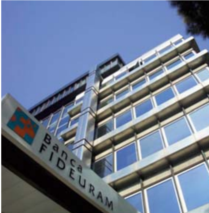
Rome, Piazzale Douhet, Registered Office
