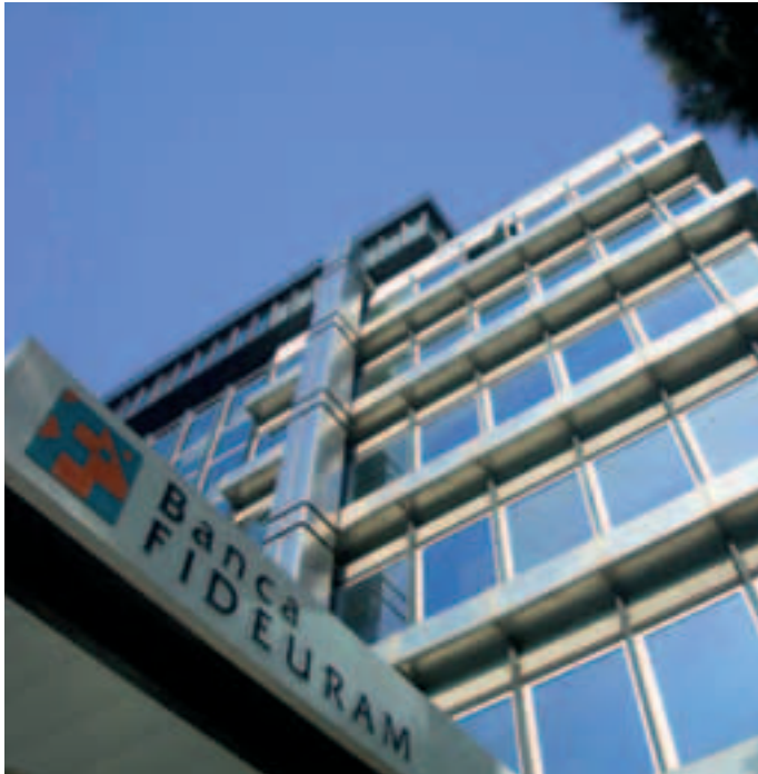
Rome, Piazzale Douhet, Registered Office
