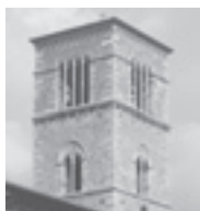
16. Terni Steeple, San Francesco Church
